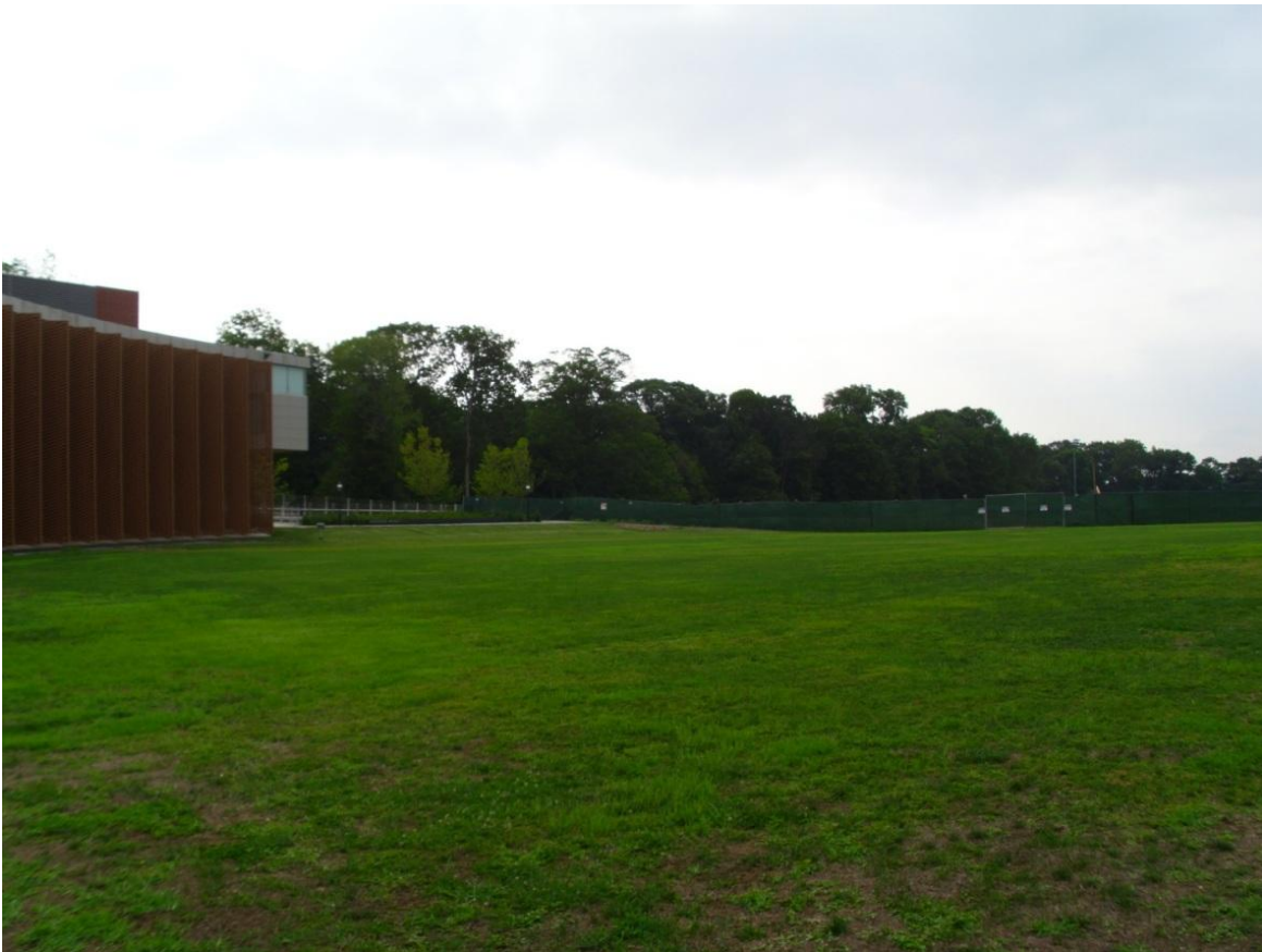
SITE UNDER CONSTRUCTION, ICAHN LAB TO THE LEFT
